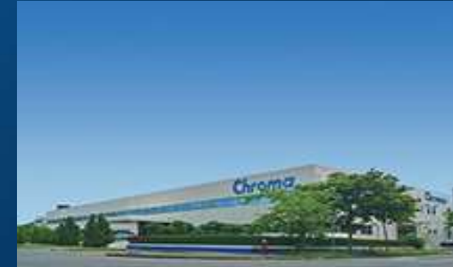
Kaohsiung Factory 13,469 m 2
