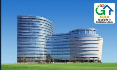
HQs & Taoyuan Factory 104,141 m 2
